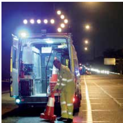
Road hazard ahead. Merge lanes.
